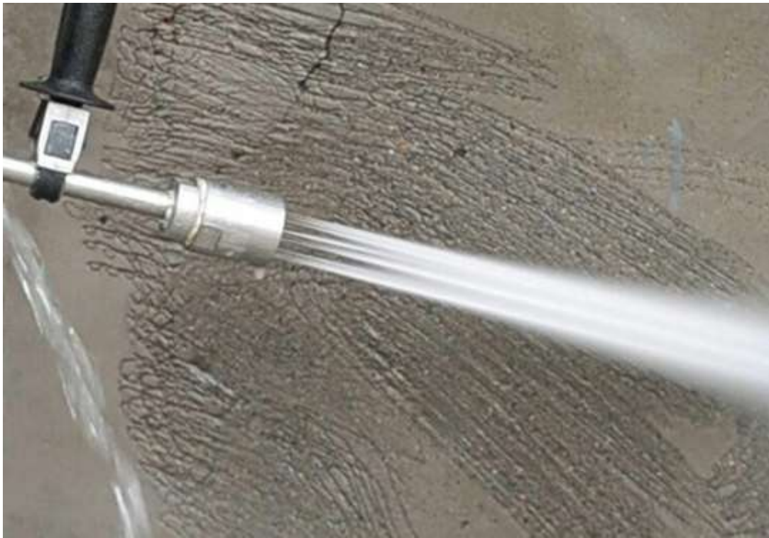
Figure 3.13 – High pressure water jet method
