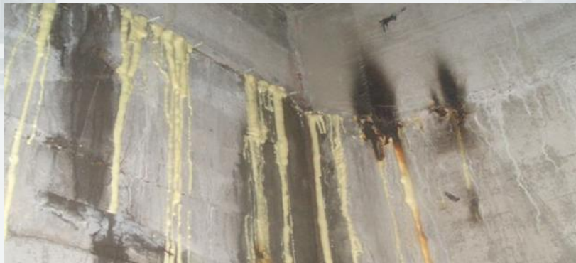
Leakage of concrete structure
