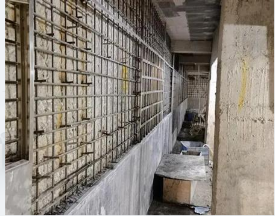
Reinforcement of shear wall
