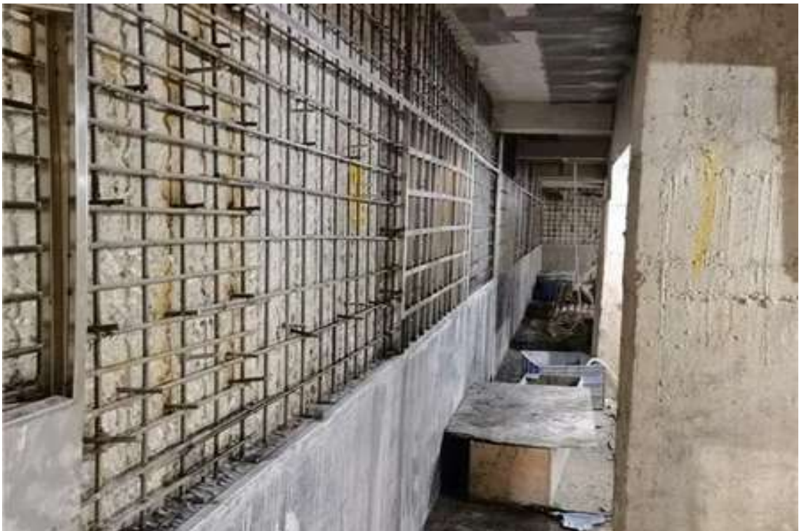
Figure 3.9 – Reinforcement of shear wall
