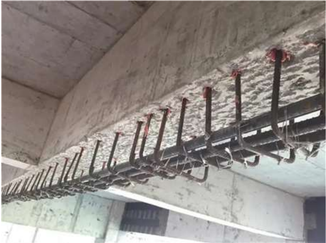
Figure 3.8 – The beam is strengthened on one side
