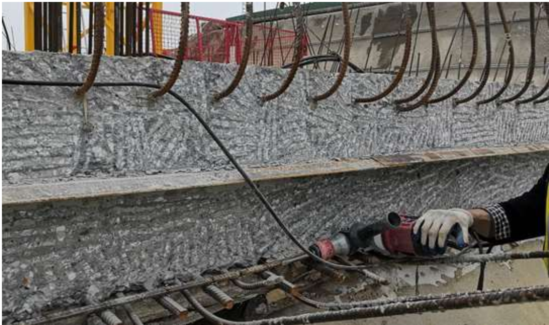
Figure 3.12 – Manual chisel method
