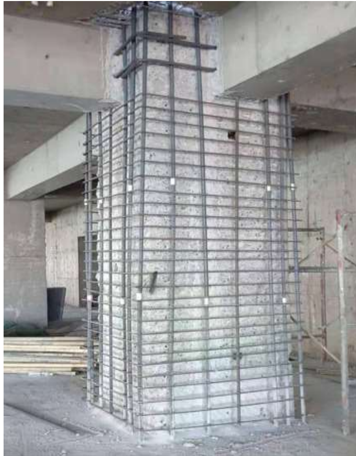
Figure 3.7 – Column reinforcement on four sides
