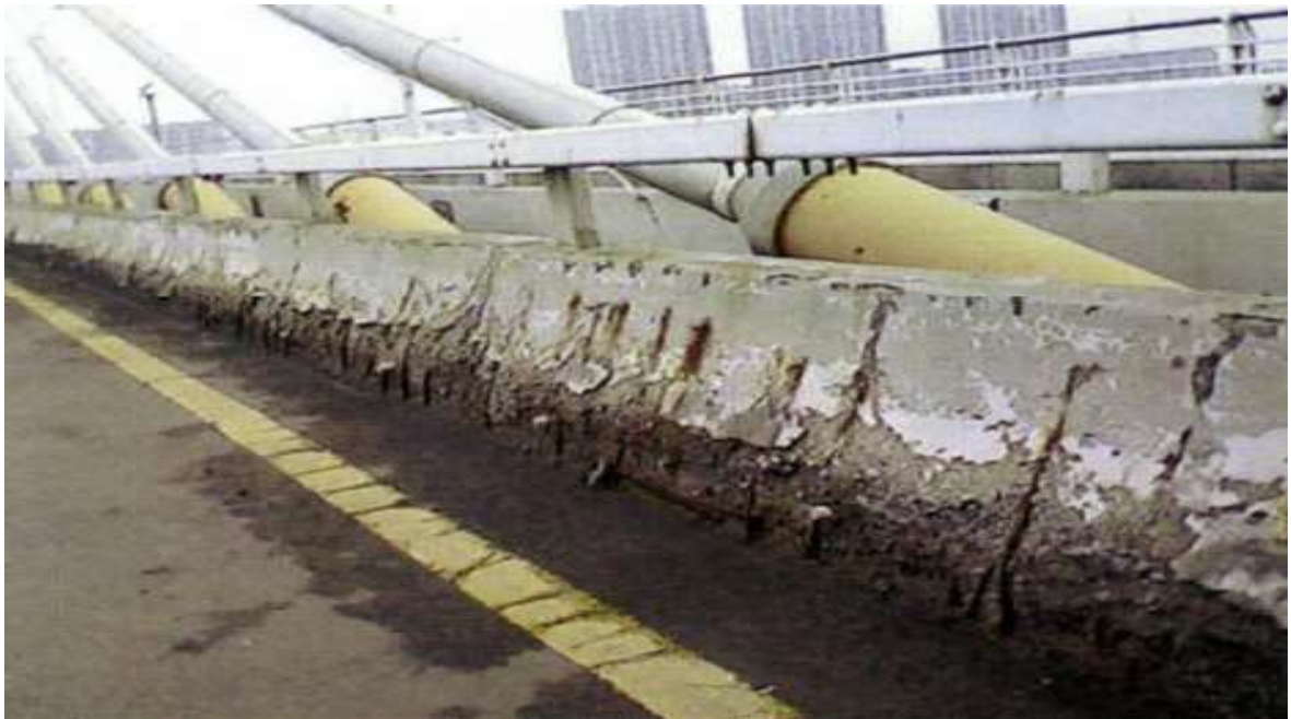
Figure 3.3 – Corrosion of concrete structure
