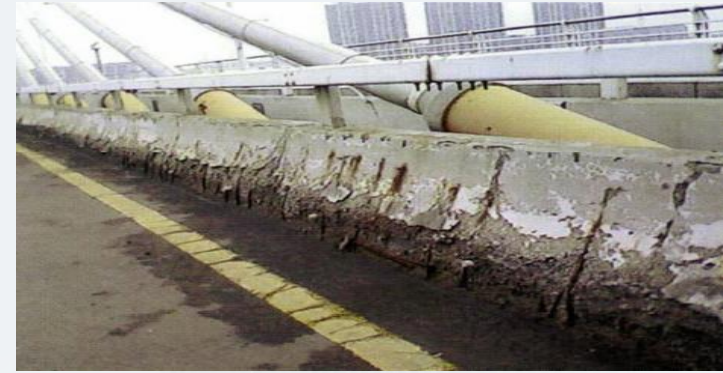
Corrosion of concrete structure
