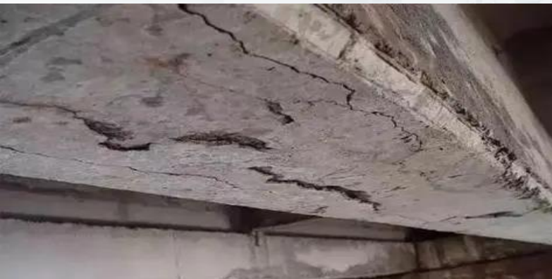
Frost heave failure of concrete structure
