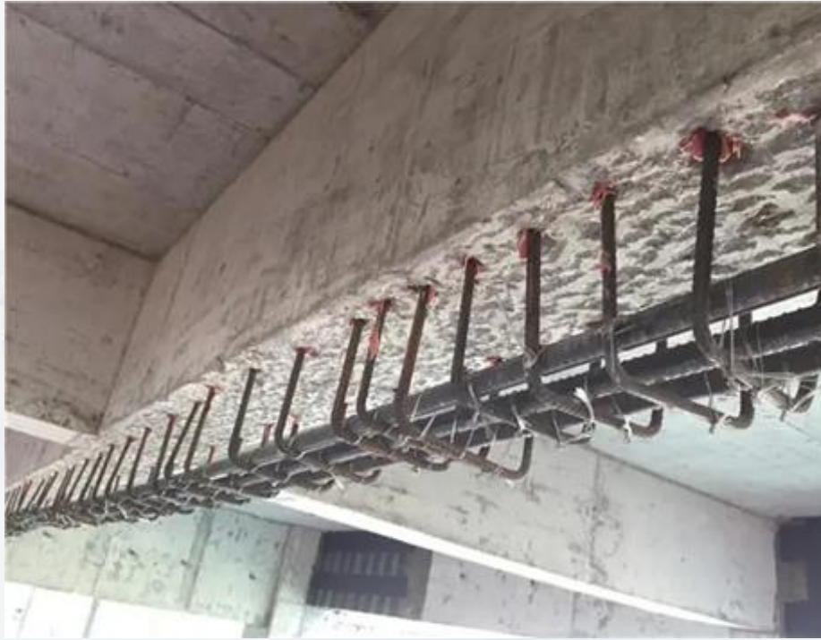
The beam is strengthened on one side
