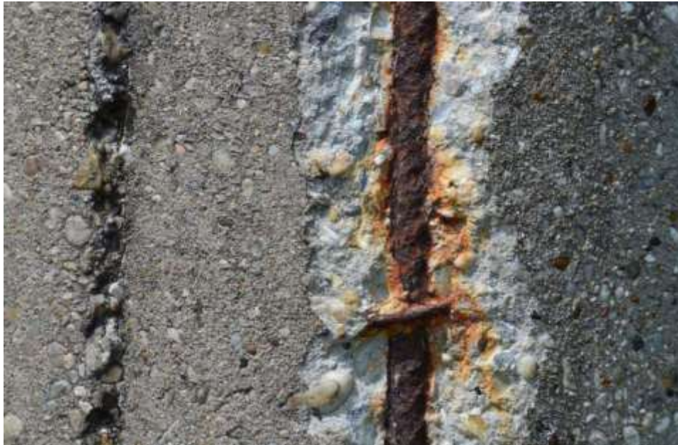
Figure 3.6-Aging of concrete structure
