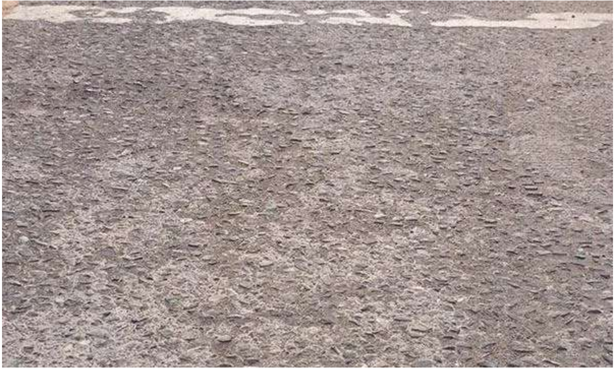
Figure 3.14 – High pressure water jet method
