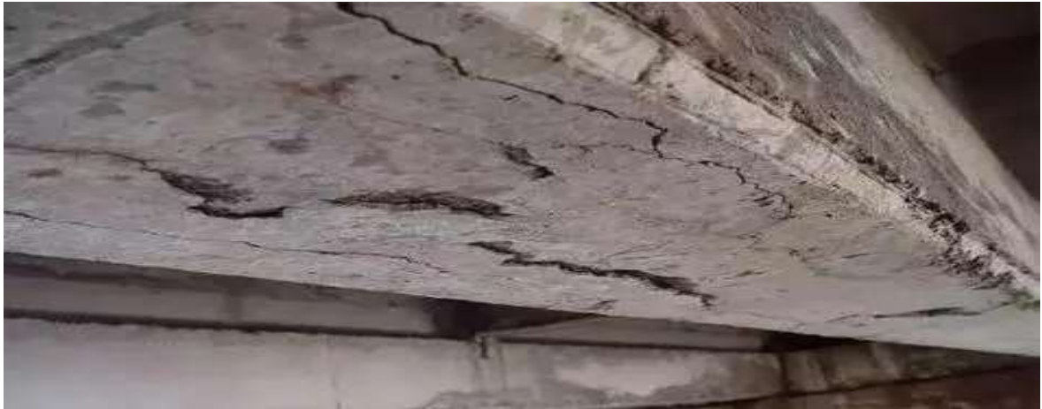
Figure 3.4 – Frost heave failure of concrete structure
