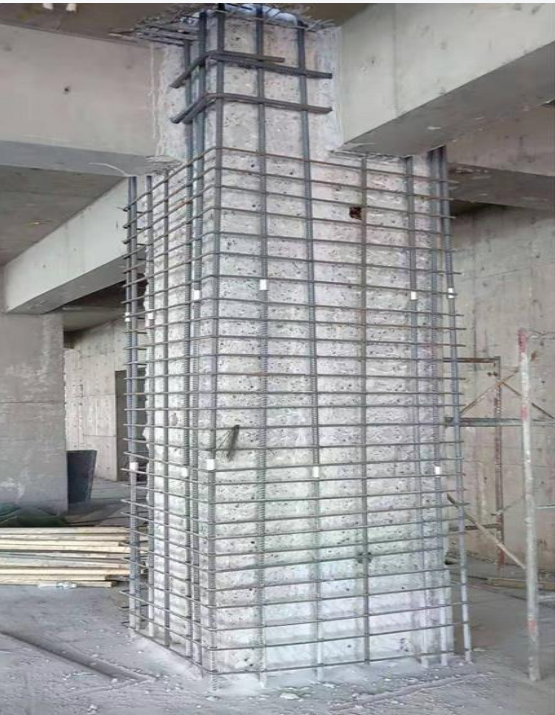
Column reinforcement on four sides
