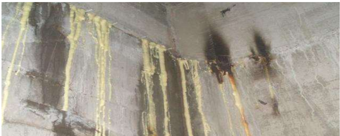
Figure 3.5 – Leakage of concrete structure
