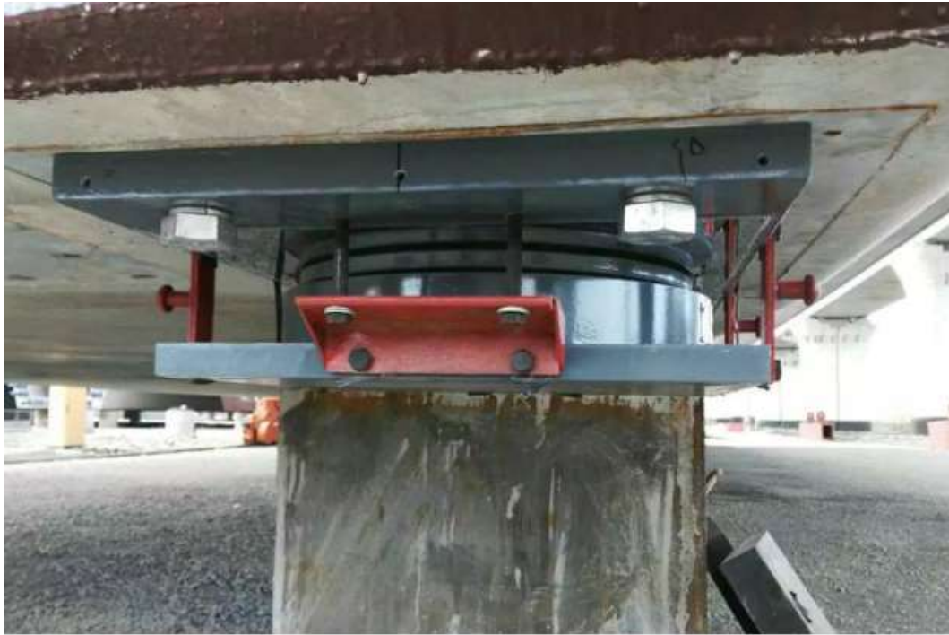
Figure 1.14 – Typical elastomer bearings for bridge support
