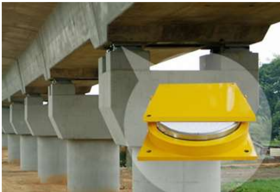
Figure 1.2 – Bridge Bearings
