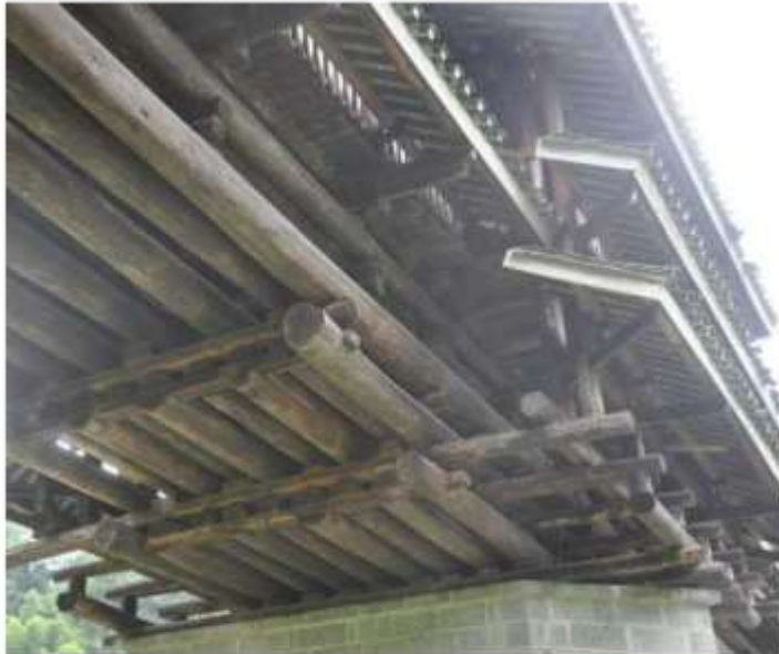
Figure 2.3 – Typical support structure of ancient Chinese bridges
