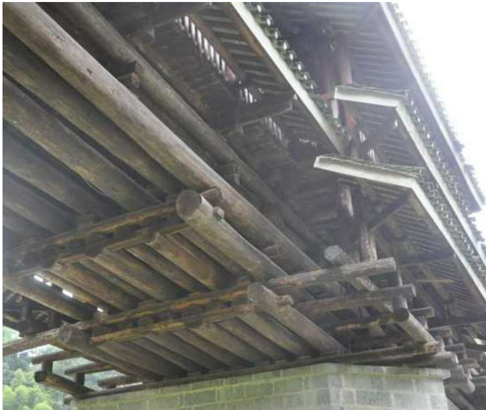
Figure 1.9 – Typical support structure of ancient Chinese bridges
