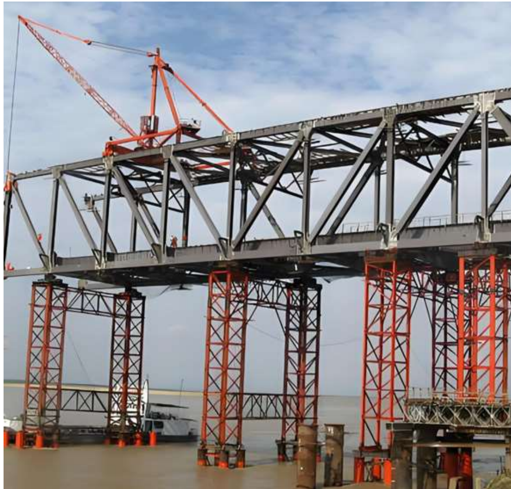
Figure 1.10 – Typical support structure of modern Chinese bridges
