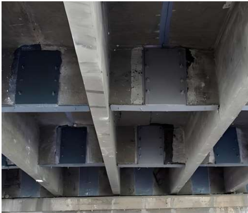
Figure 1.5 – Multi-layer support with beams
